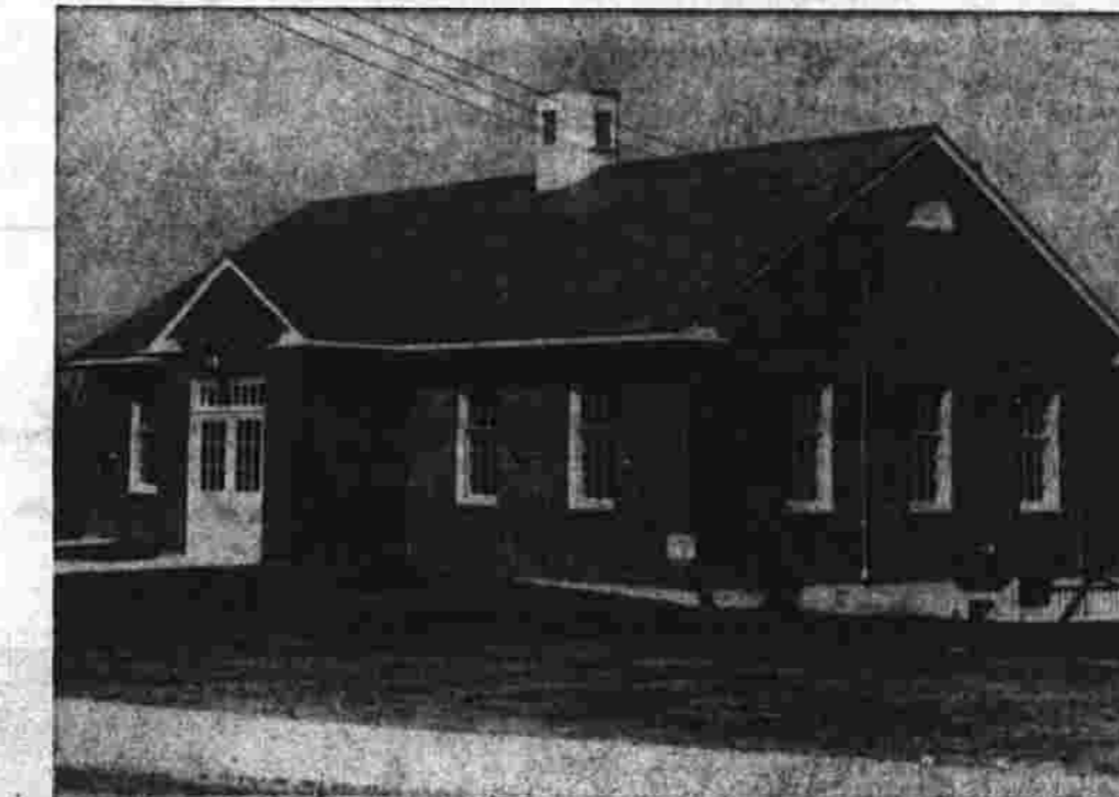
We are proud that we were selected to build this new structure, designed to harmonize with the YMCA and Whiton Library. We extend our best wishes to the officers and directors of the Manchester Trust Co. for their continued success.
